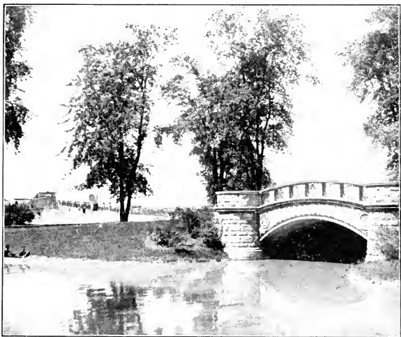
Entrance to Belle Isle from the Bridge.
